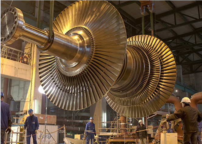
Servicing a Mitsubishi Power steam turbine
