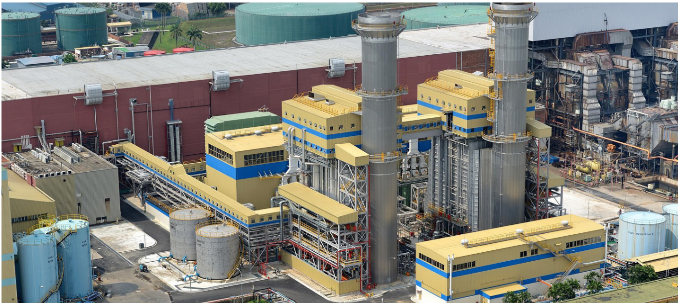
Senoko Energy GTCC Power Plant
